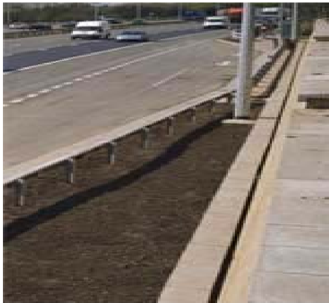
An emergency refuge area
